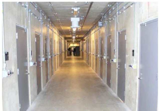
Secure underground bunker security
